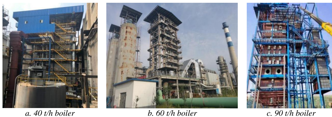
Figure 3: Industrial application of coal self-preheating combustion technology
