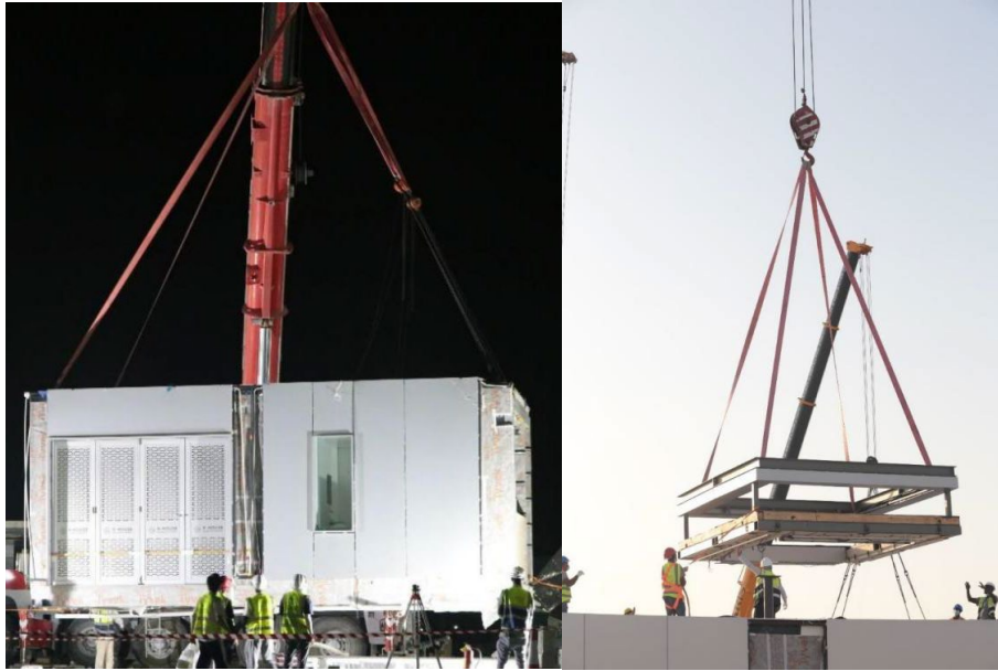
Figure 6: Module Unit Lifting, Roof Unit Lifting
