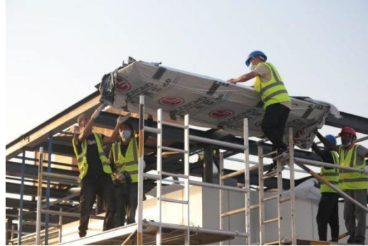
Figure 8: Installation of roofing elements
