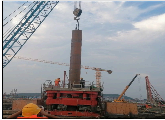
Figure 4: Real-time Correction of Steel Casing Sinking Verticality
