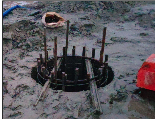
Figure 6: Hoisting of Reinforcement Cages
