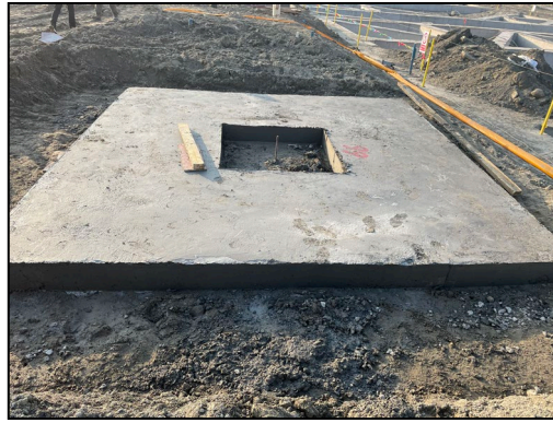
Figure 2: Site Leveling and Hardening
