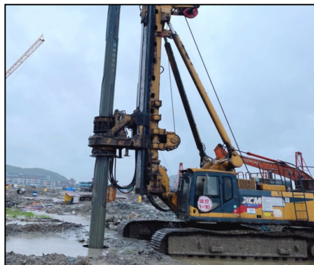
Figure 5: Formation of Bored Piles with Rotary Drilling
