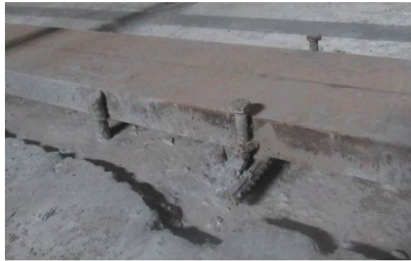
Figure 4: Fine-Aggregate Concrete Pouring for T-shaped High-Precision Embedded Parts
