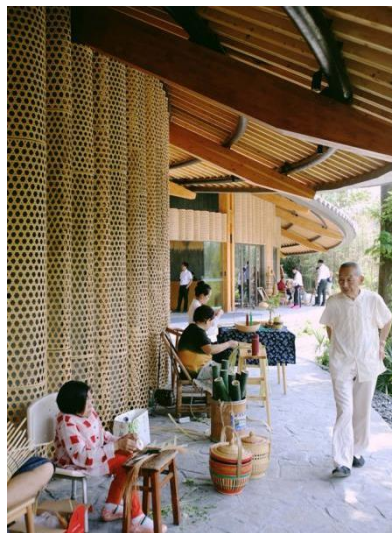
Figure 3: The bamboo mold concrete wall
