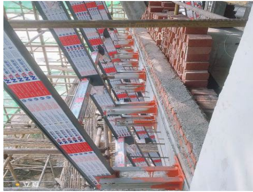
Figure 3: Art Center Keel Installation
