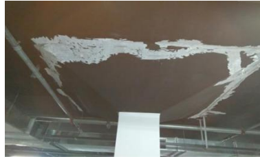
Figure 1: Photograph of lateral cracks in column cap
