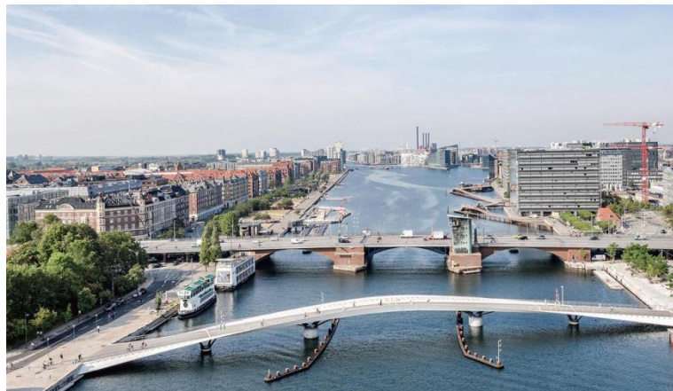
Figure 3. The bicycle viaduct in Copenhagen
