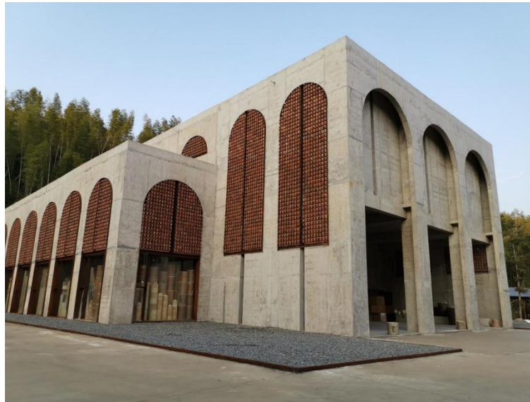
Figure 2: The external space of Bingding wood-fired kiln
