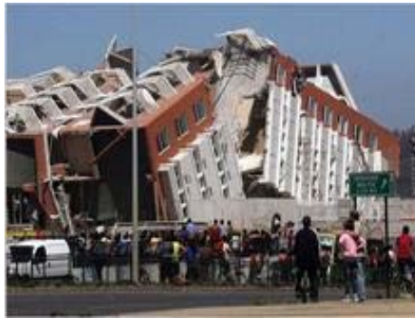
Figure. 1 Collapse caused by column hinge mechanism
