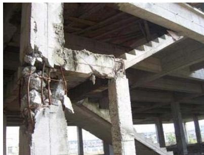
Figure. 4 Short column formed at the landing
