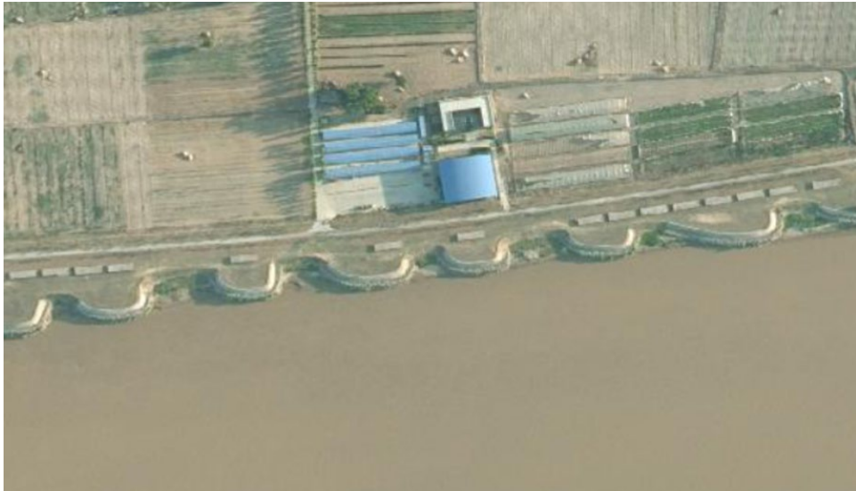
Figure 3: Phenomenon of disorderly construction and occupation
