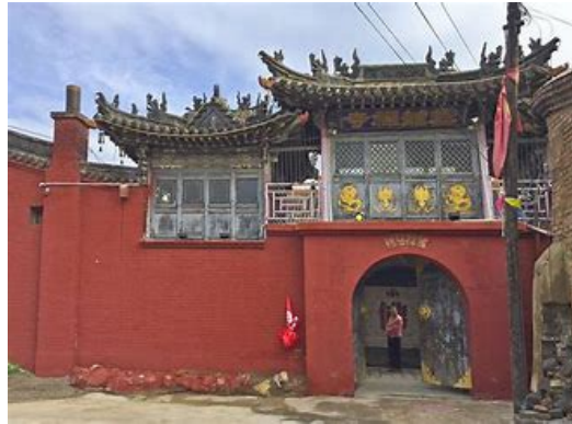
Figure 3: The situation around Datong ancient City Wall.
