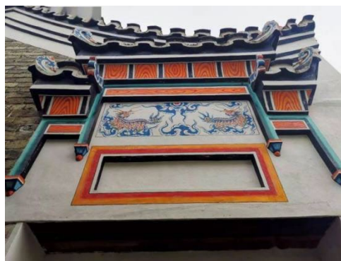
Figure 7: Xidi Village Paint at will.
