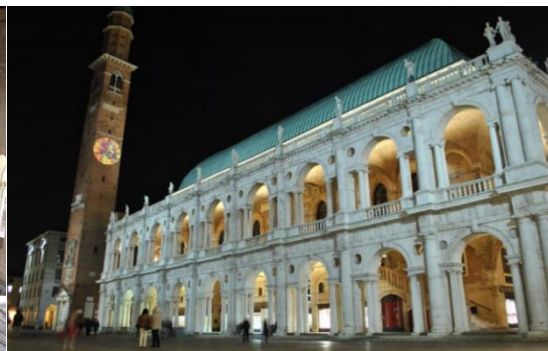
Figure 7: The present facade of the building.
