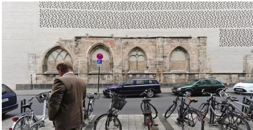
Figure 15: The combination of the new building and the heritage.
