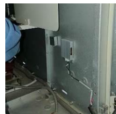
(b) Ultrasonic sensor and heater installation.
