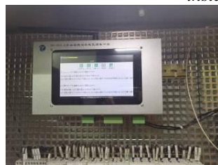
(e) Concentrator installation.
