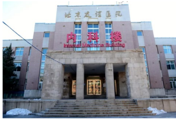
Figure 3: Youyi Hospital Outpatient Building
