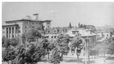
Figure 5: Tongren Hospital Complex
