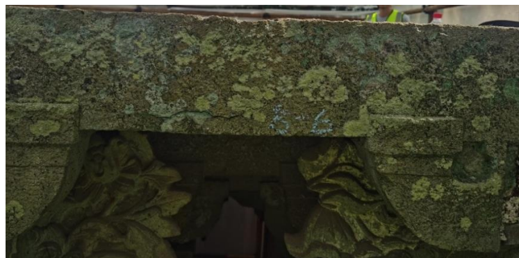
Figure 3: Surface of mortise and tenon of No.6 on the south side of the top of Bai Goose Pavilion in Tianyi Pavilion
