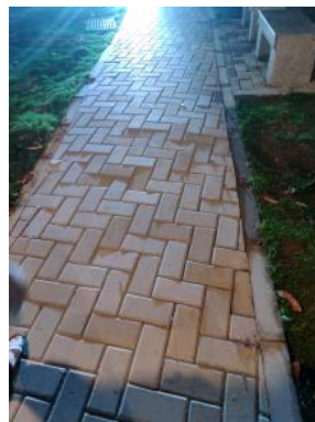
Figure 2 Road conditions of Henanan Park
