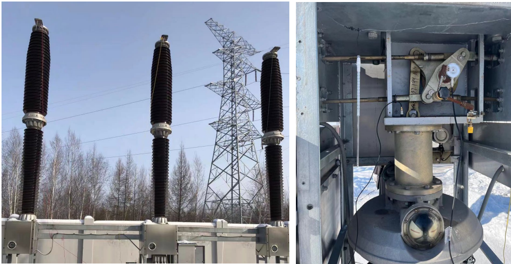
Figure 1: SF 6 circuit breaker and operating mechanism
