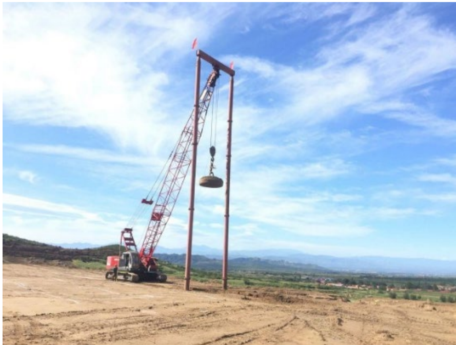
Figure 1: Dynamic compaction method
