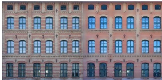
Figure 9: Façade before and after comparison
