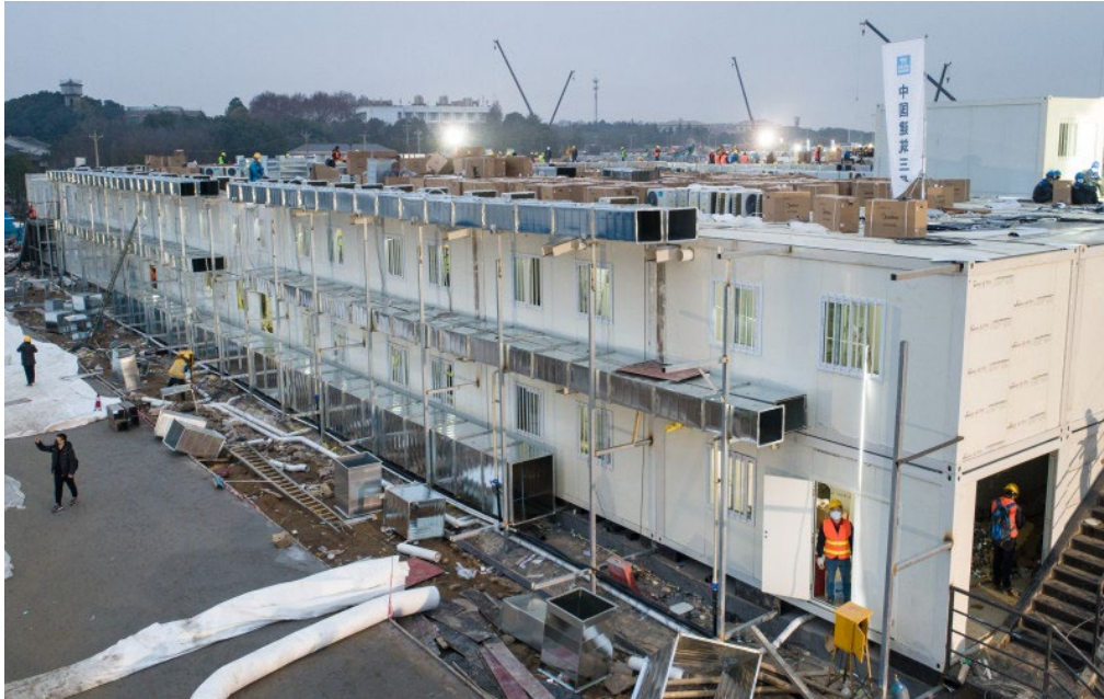
Figure 1 Modular Construction Diagram of Wuhan Huoshenshan Hospital
