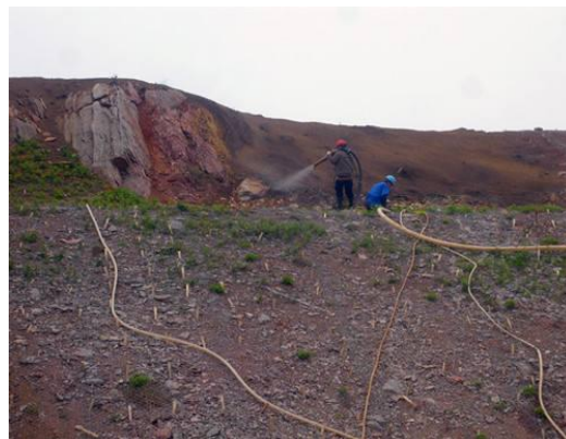
Figure 3: The technology of net-hanging spray-broadcasting
