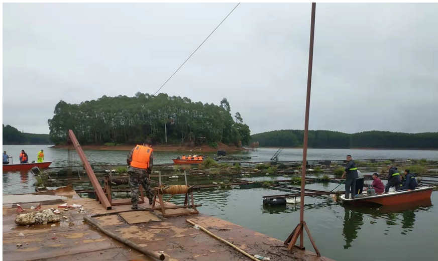
Figure 1: Cleaning illegal cages in Pubei Reservoir
