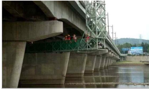
Fig. 2 Inspection workers standing on temporary scaffolding
