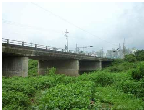
Fig. 3 View of the Amsogogae Bridge
