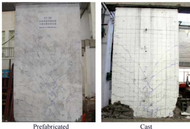
Figure 20. Development of crack in shear wall
