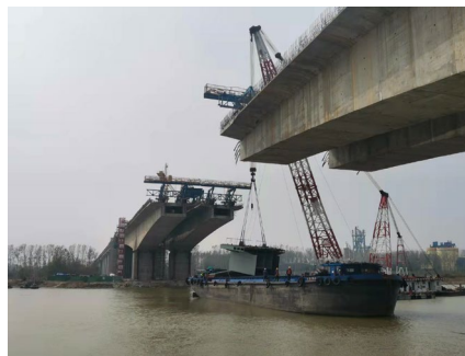
Figure 5: Lifting of the steel-concrete composite segment by the floating crane
