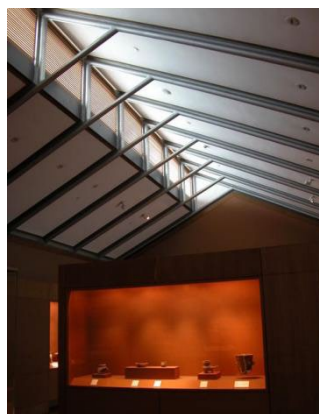
Figure 5: Interior structure with light introduced
