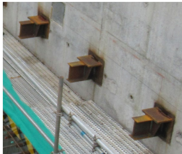
Figure 1: Steel Corbel Installation
