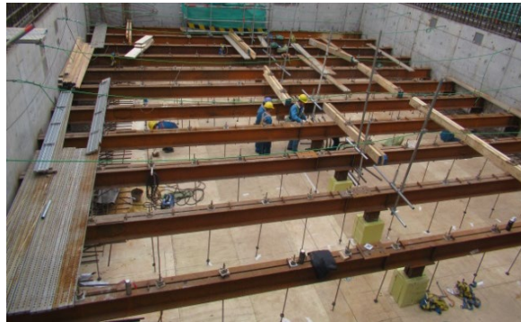
Figure 3: High-Strength Tie Rod Installation
