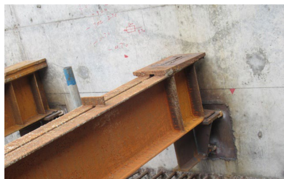
Figure 2: Installation of Steel Beam to Steel Corbel Connection
