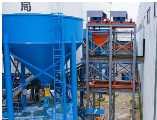
Figure 3: Concrete hoisting system.
