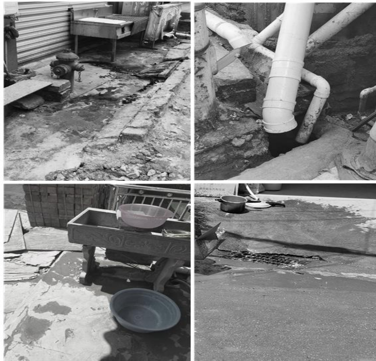
Figure 1: Current status of sewage collection in Sikouzun Village.
